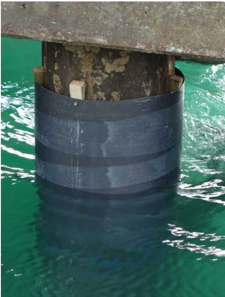
Figure 5: FRP jacketing of Boatlift structure timber pile
