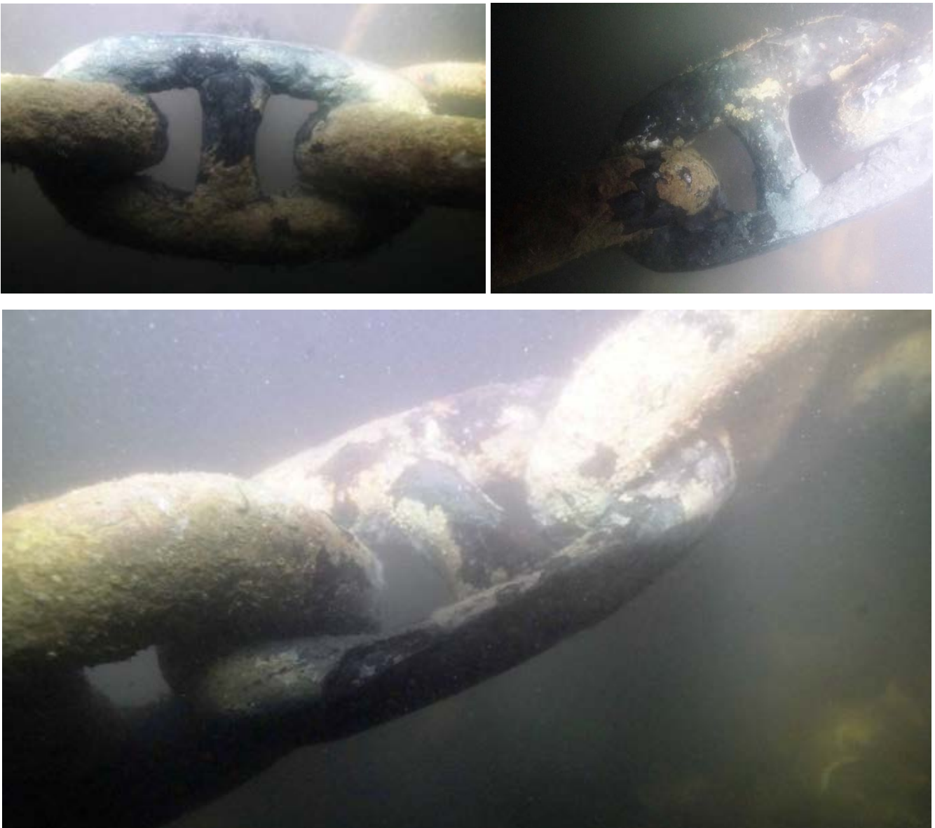
Figures 22, 23 & 24: South-leading ground chain – temporarily elevated out of seabed with use of a Lift-bag. It's believed that due to dredging when the OPT was operating, the seabed was reduced down to where a tight bound sedimentary layer of shell and stone composition now immediately underlies the current shallow mud and silt layer. This material is proving to be quite aggressive on the mooring chains within and beyond the thrash zone. With the correct pretension now being applied to the moorings, and subsequently minimised movement in Station, the affected zone should be significantly reduced
