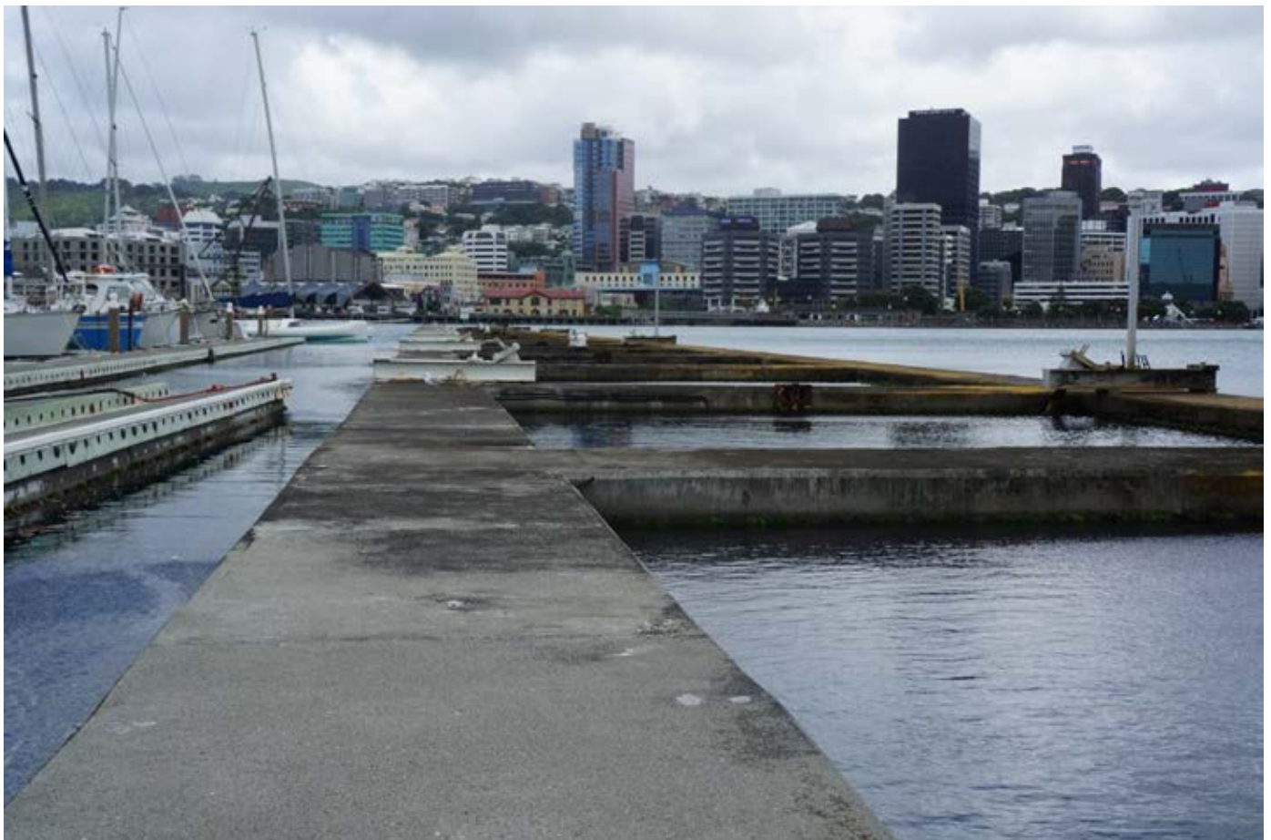
Figure 1: Chaffers Marina floating concrete breakwater
